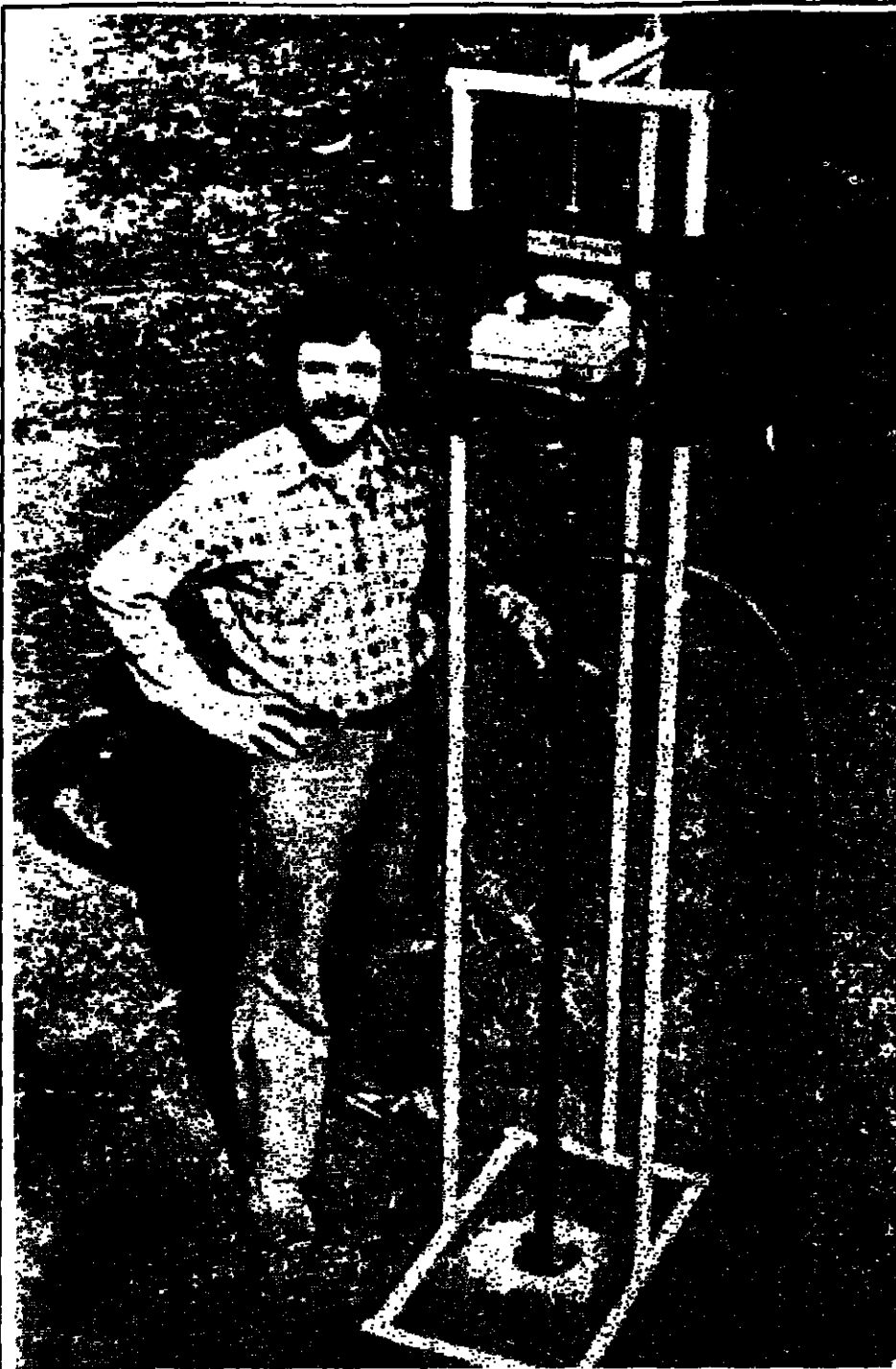
DRILL YOUR WELL: Hydra-Drill, a do-it-yourself technology in well drilling is a portable kit produced in Alabama, USA, the unit drills small diameter (5 cm) wells up to a maximum depth of 60 meters. The wells can produce as much as 400 gallons per hour pumped by hand, windmill, gasoline or electric pump.
